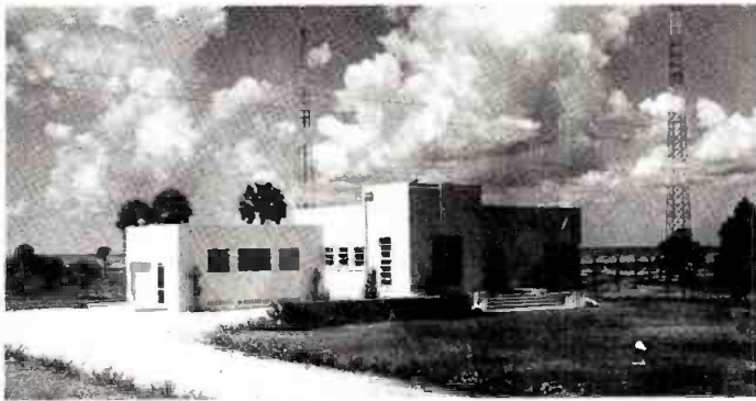
Modern Transmitter House
